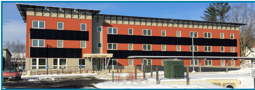
The building features photovoltaic panels on the roof, cornice, south-facing facade, and a solar arbor
